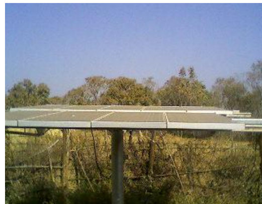
Figure 58 – Decentralized application of solar power for pumping water in Melghat, a tribal village
